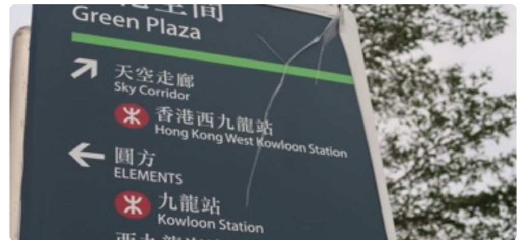
Signs peeling off from the newly constructed West Kowloon High Speed Rail Station.
